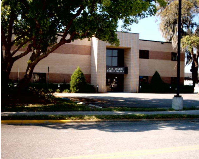
Lake County Public Works Building
