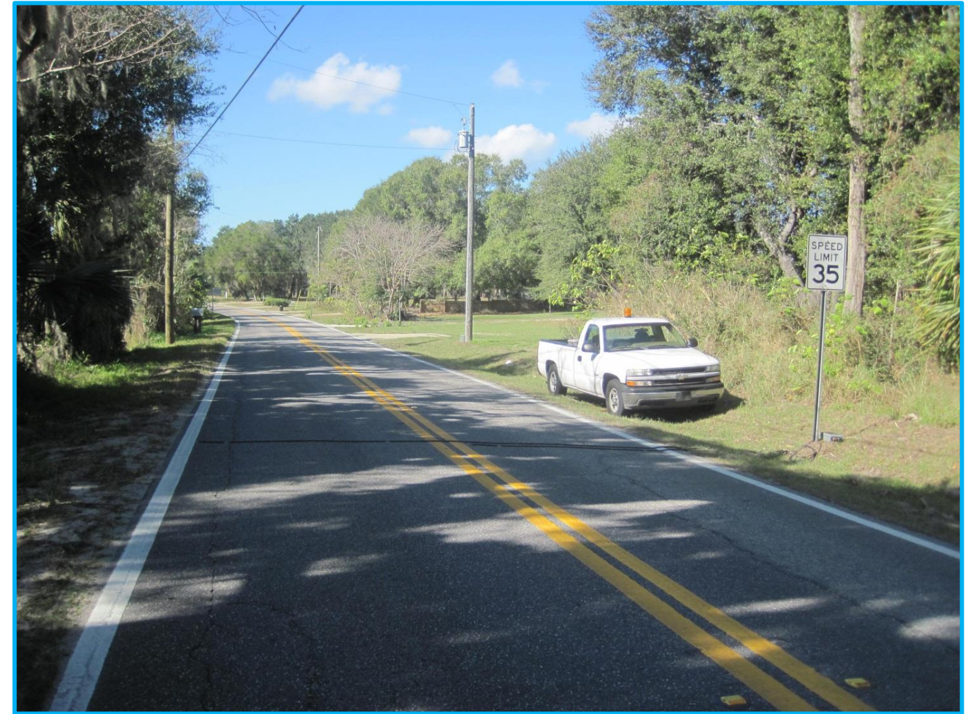
Typical view of Lake County Annual Traffic Count Station setup
