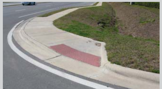
View of curb ramp with detectable warning looking west towards proposed bus stop location
