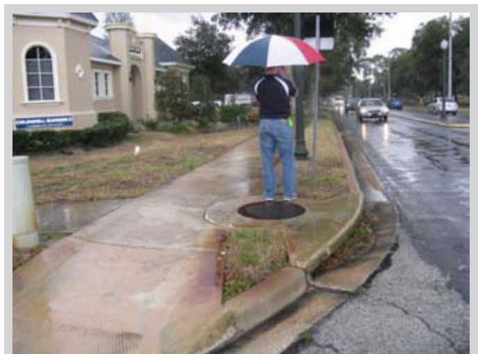
Current view of bus stop looking south.
