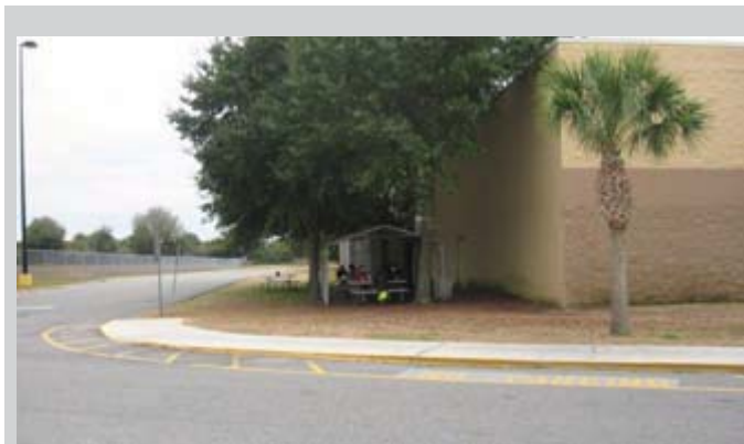
Current view of bus stop looking south
