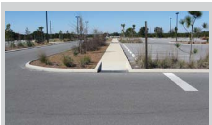
Accessible path from park to bus stop travelling west
