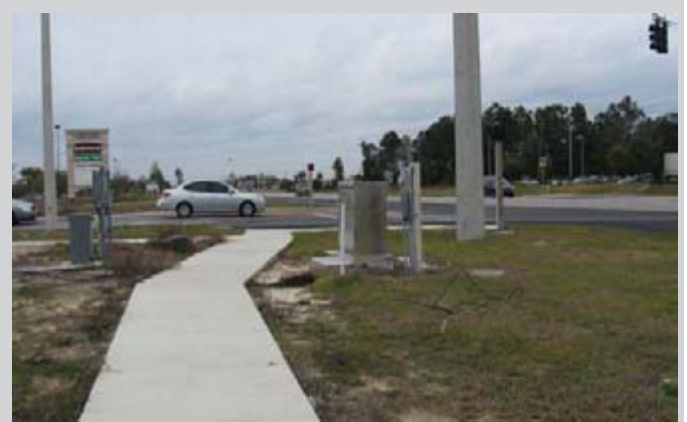
Current view of sidewalk looking west
