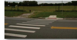
A crosswalk exists over SR 471 in front of Webster Elementary School.
