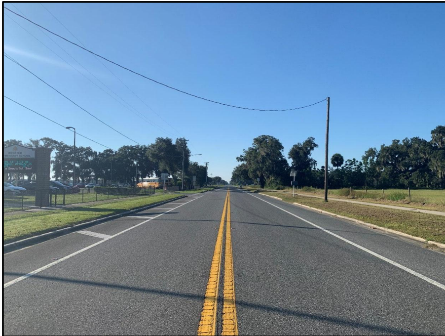
Looking south from the crosswalk along SR 471 (S Market Boulevard)
