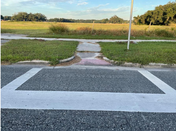
Photograph 13: Existing crosswalk curb ramp on western side of road in front of Webster Elementary School
