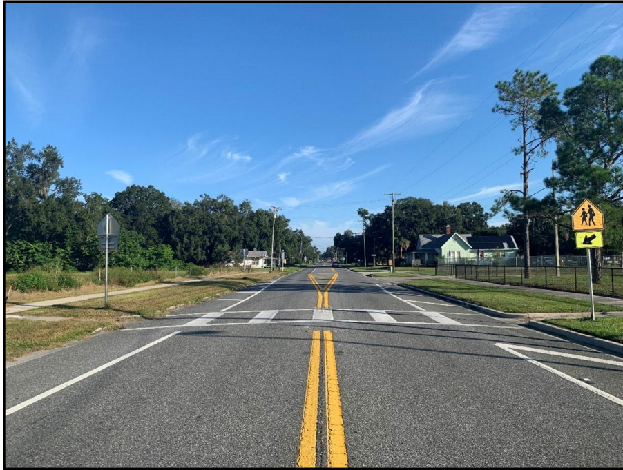
Looking north into the crosswalk along SR 471 (S Market Boulevard)
