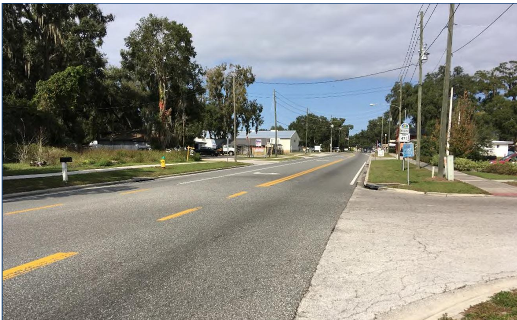
SR 471 & CR 478 - looking north
