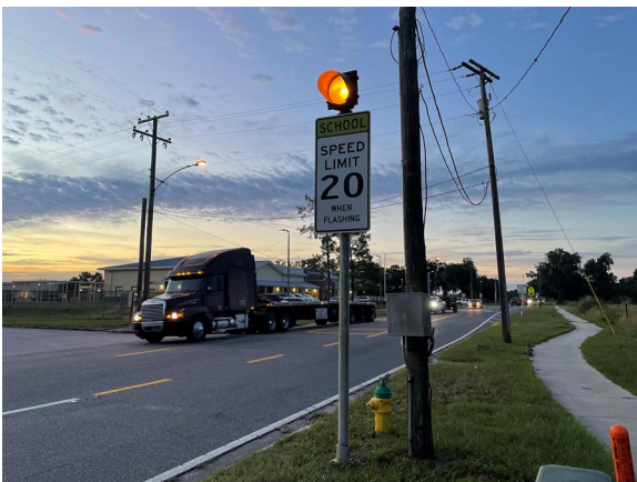
Photograph 17: Flashing school zone sign north of Webster Elementary School on SR 471
