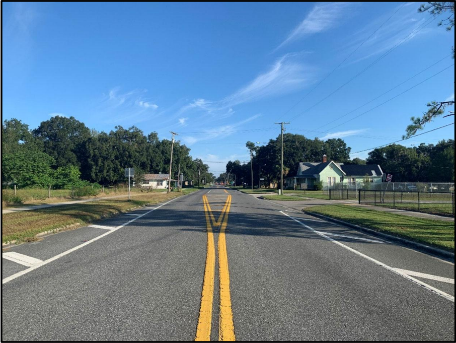
Looking north from the crosswalk along SR 471 (S Market Boulevard)
