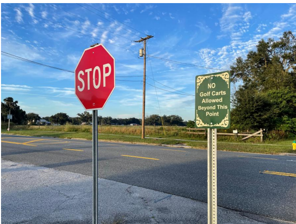
Photograph 11: SR 471—facing east from SE 3 rd Avenue
