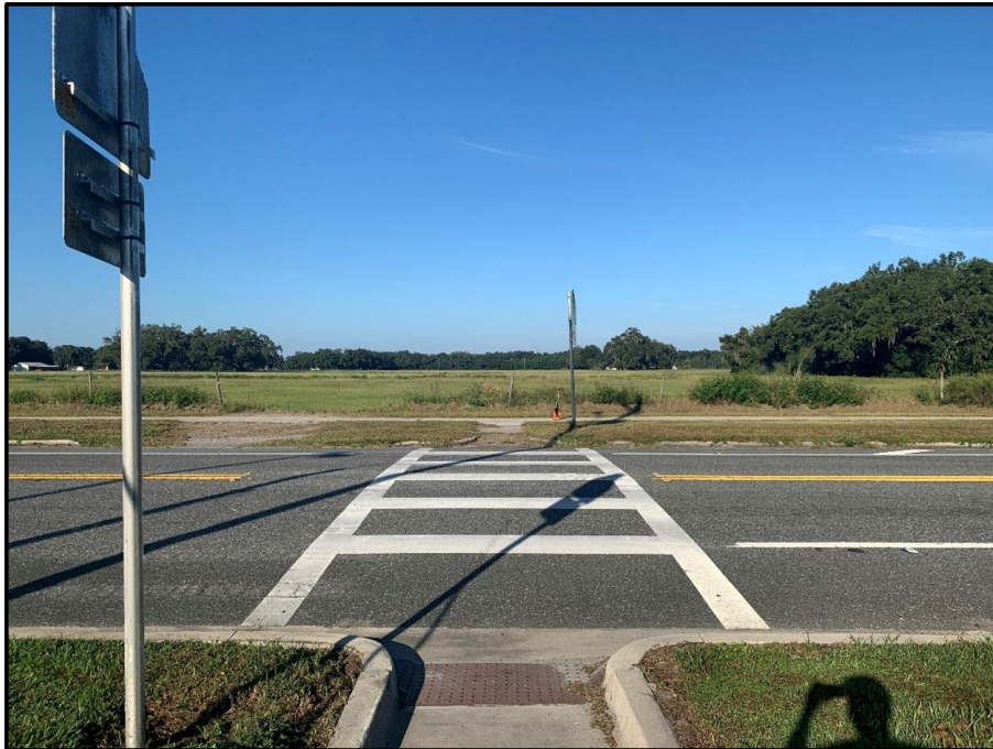
Looking west into the crosswalk at Webster Elementary School
