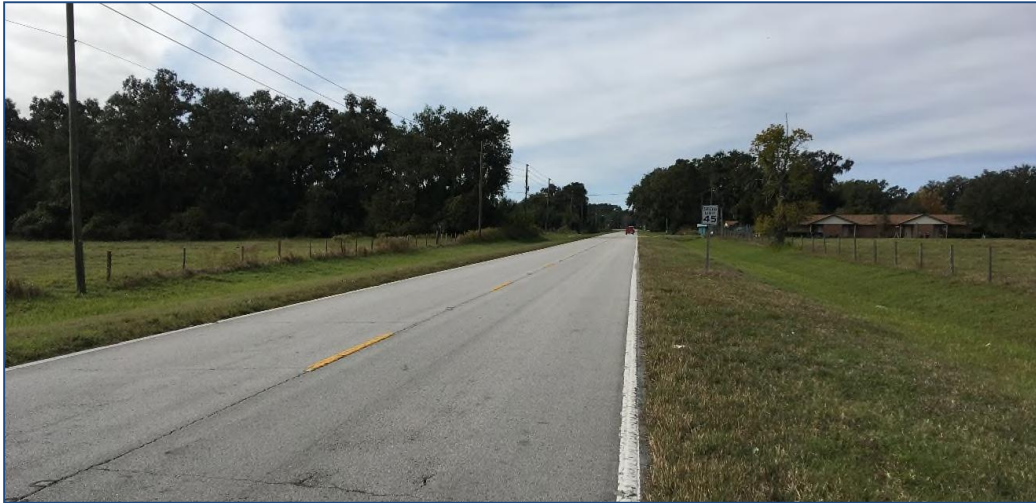
CR 478 & Project Access - looking west
