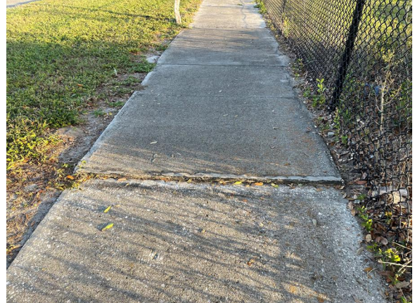
Photograph 14: Existing sidewalk in front of Webster Elementary
