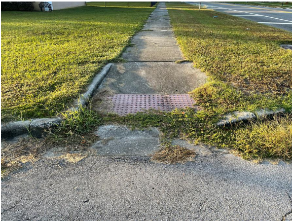
Photograph 21: Existing southern curb ramp at the intersection of SR 471 SE 2 nd Avenue
