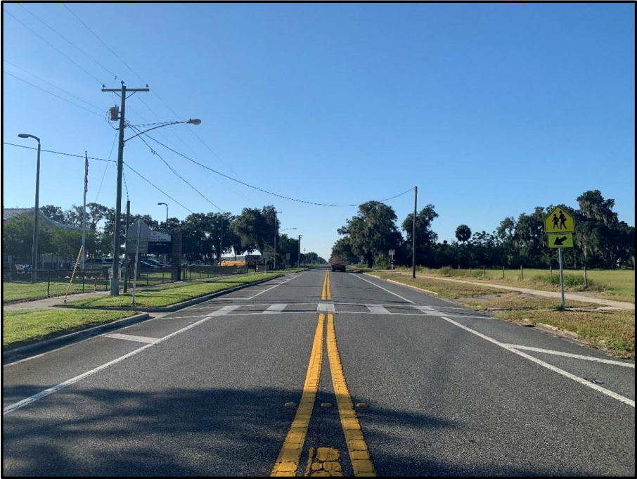
Looking south into the crosswalk along SR 471 (S Market Boulevard)
