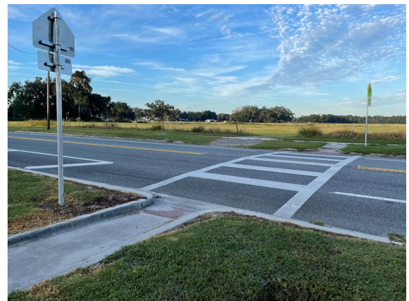
Photograph 12: Existing crosswalk in front of Webster Elementary School
