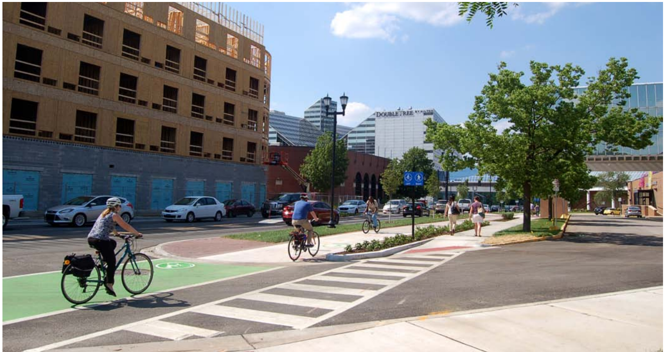
Smart Streets improvements on St. Joseph Boulevard. Photo courtesy of City of South Bend.
