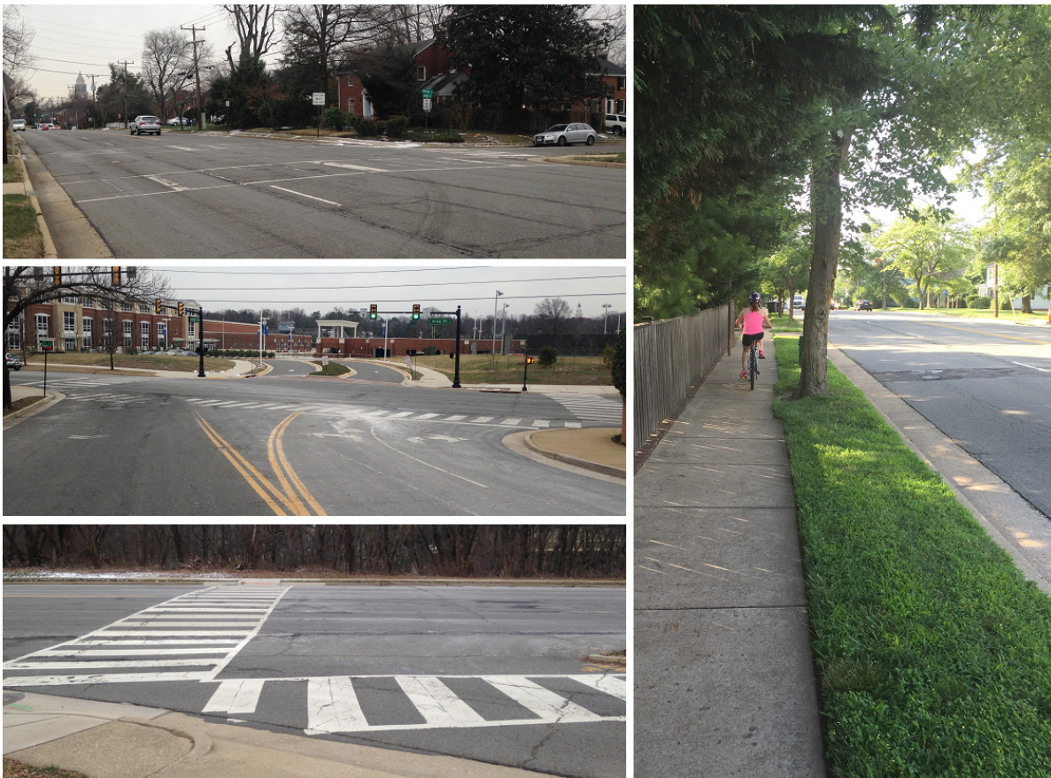
King Street before Complete Streets improvements. Photos courtesy of City of Alexandria.
