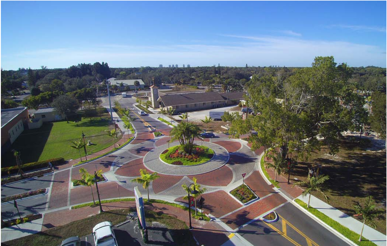
Aerial view of new roundabout. Photo courtesy of City of Bonita Springs.
