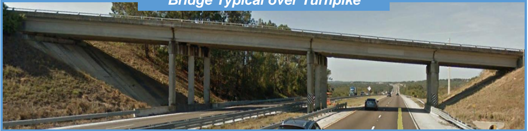
Existing Scrub Jay Lane Bridge Typical over Turnpike
